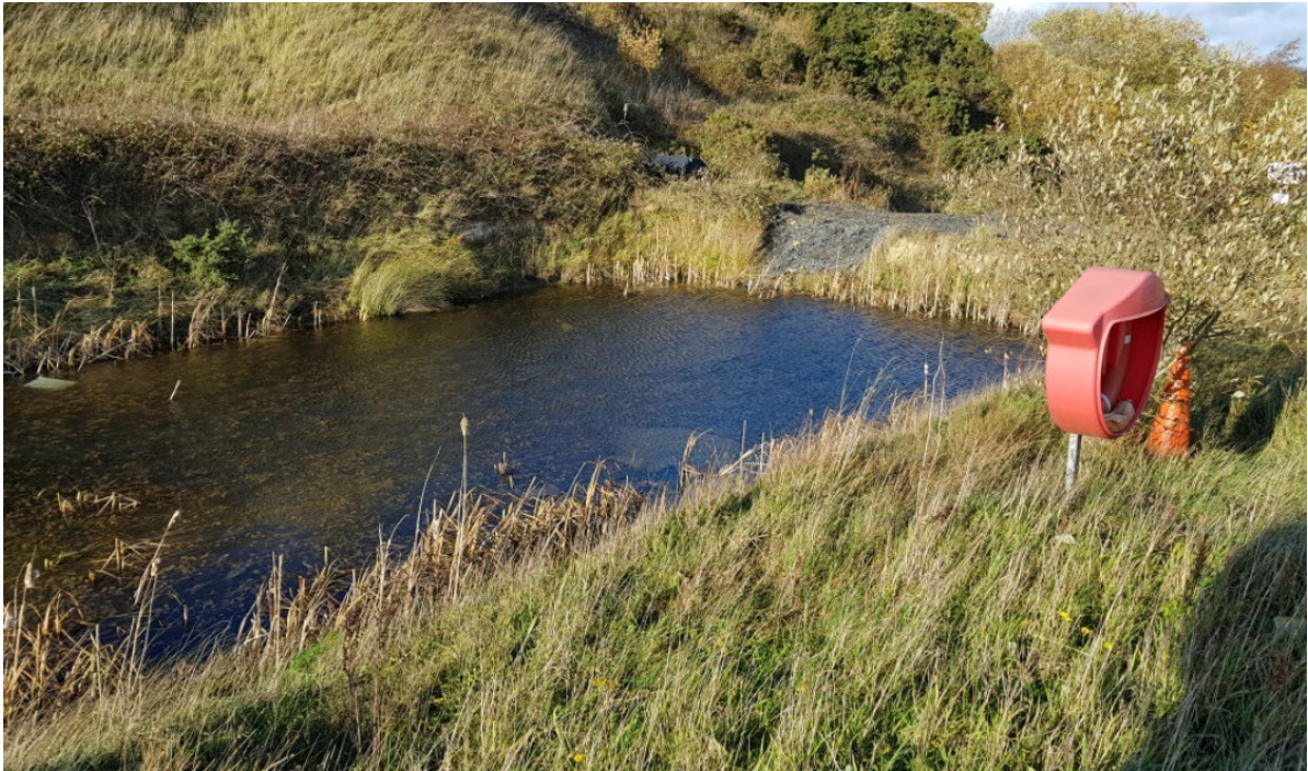
Figure 18: Settling Pond 1 (Overflow Pipe Below Water Level)
